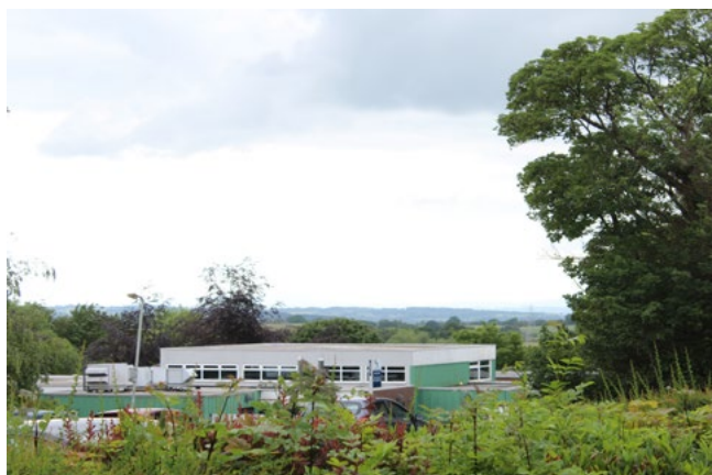
Figure 32 The flat roof of St Bartholomew's Primary School minimises its impact upon views out of the Conservation Area
