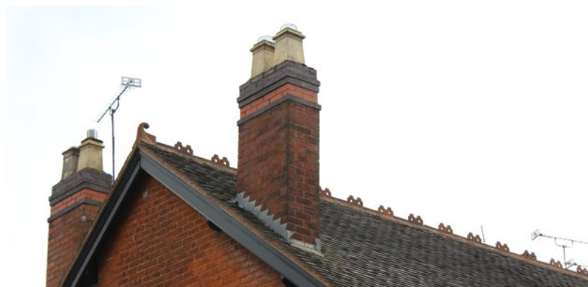
Figure 24 Decorative ridge tiles provide visual interest to the skyline
