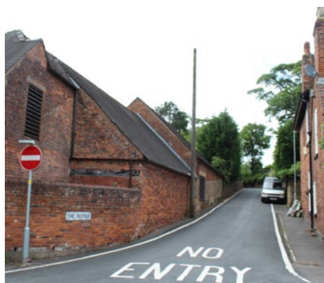
Figure 34 Unsympathetic signage detracts from the rural character of The Avenue
