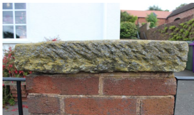
Figure 22 Stone Copings on brick walls provide visual interest
